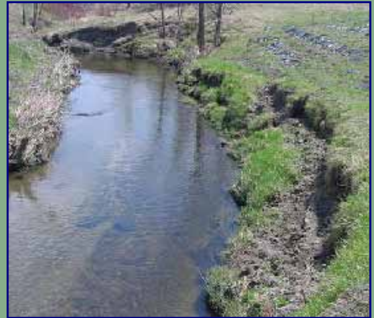
Eroded shoreline with exposed roots and soil
